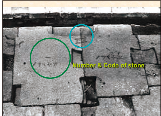
Numbering and coding on stone block before dismantling
