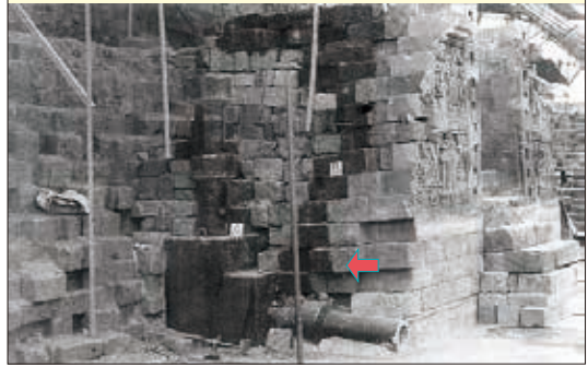
Concrete pipe construction
