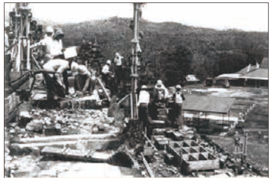
Dismantling of gallery floors are cemented with mortar
