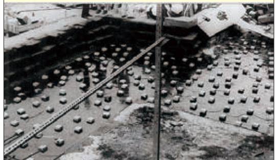
Reinforcement concrete foundation
