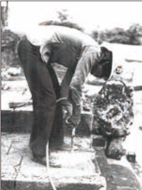
Numbering and coding on stone block before dismantling
