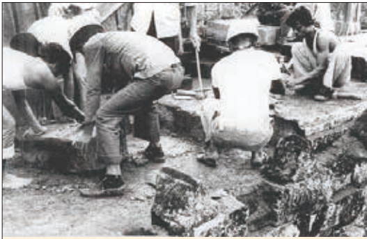
Dismantling of stone blocks
