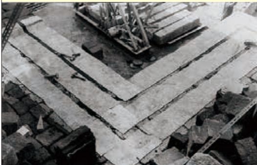
Construction lead coating
