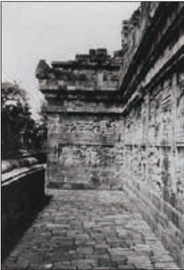
Gallery floor after repairing
