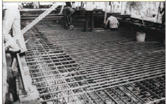
Reinforcement concrete foundation
