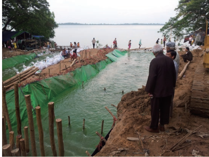
Figure 5.2.3: Urgent intervention at Ancient Spillway during the flood 2013 to reduce water pressure on West Baray dikes to save heritage (Baray) and local people's life in southern of Baray
