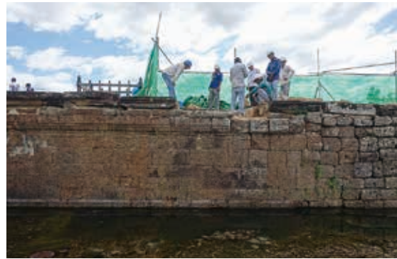
Ph. 4 Wall of laterite blocks at the area of trench 01: Grid 79-82, view from north, moat side)
