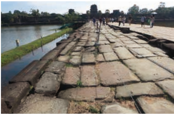
Ph. 10 Floor of sandstones, before removal
