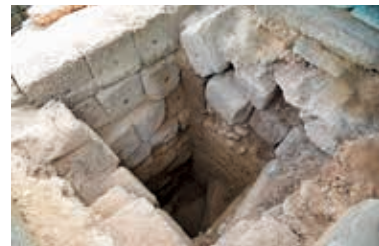
Ph. 6 Test trench 01, view from south-west
