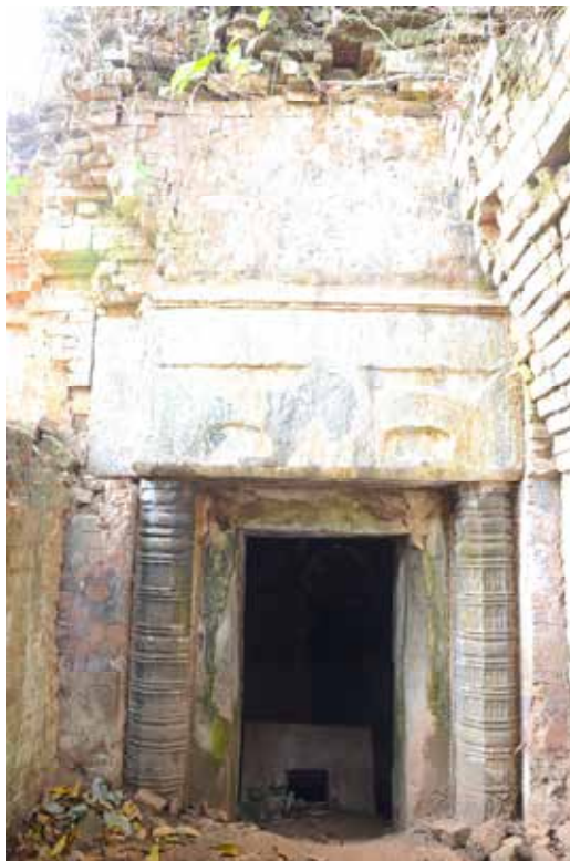
Fig. 37. Main sanctum with unfinished lintel and pediment decorations
