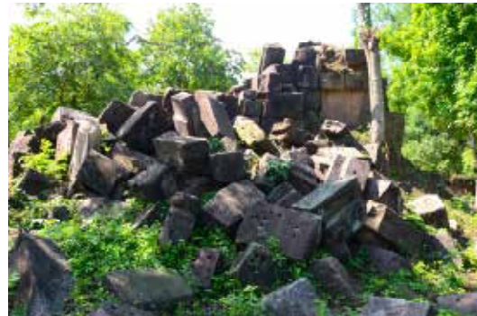
Fig. 57. Fallen apart of the temple structure
