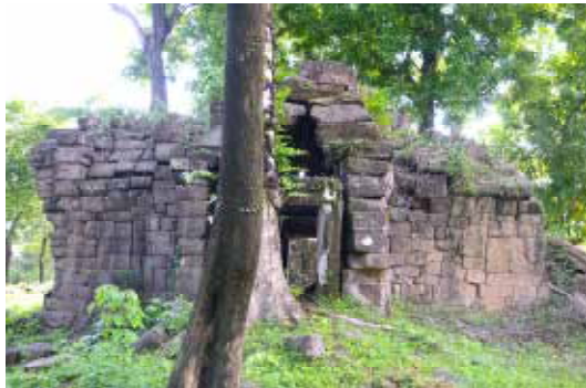
Fig. 56. A remained Gopura structure
