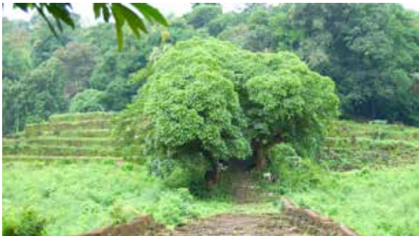
Fig. 69. Seven laterite retaining wall
