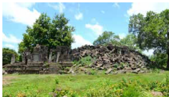
Fig. 61. Collapsed structure of the main sanctum
