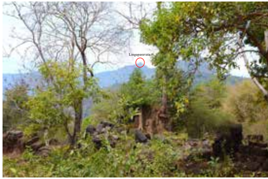
Fig. 54. Collapsed structures of sanctum and enclosure
