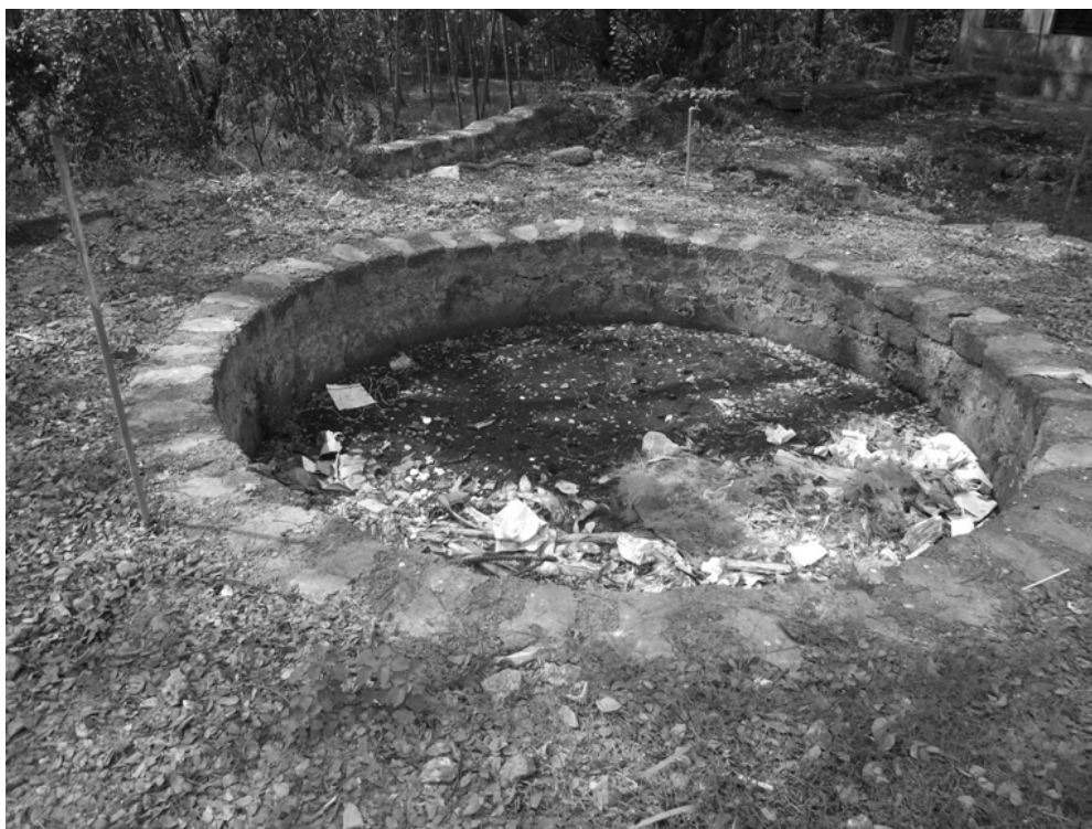
Picture-11 Covered well at St. Cajetan's Church
