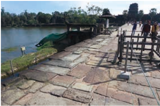
Ph. 3 Floor of sandstones, before removal
