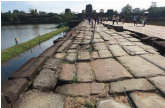
Ph. 10 Floor of sandstones, before removal
