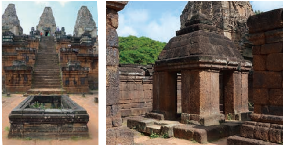
Ph. 32&33 Pre Rup temple shows the pedestal and northeast corner laterite tower
